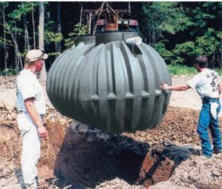
Set tank in hole and move the tank back and forth to settle tank in the gravel mixture. Use 3/8" - 3/4" gravel type aggregate.
