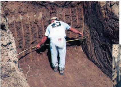
Dig and measure for appropriate tank. Allow for an extra 6-12 inches of space around the tank. Maximum depth of bury is 24" from top of tank to finish grade.
